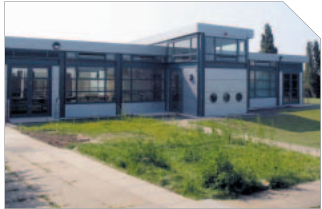
Steel Framed Volumetric Classbases at St Andrews J & I School, Colchester, Essex.
