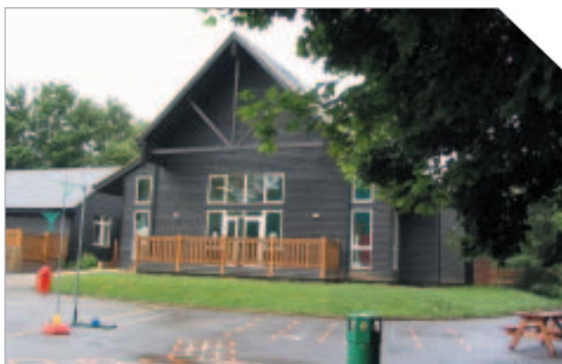
Timber Panel System Hall at Rickling Primary School, Essex.
