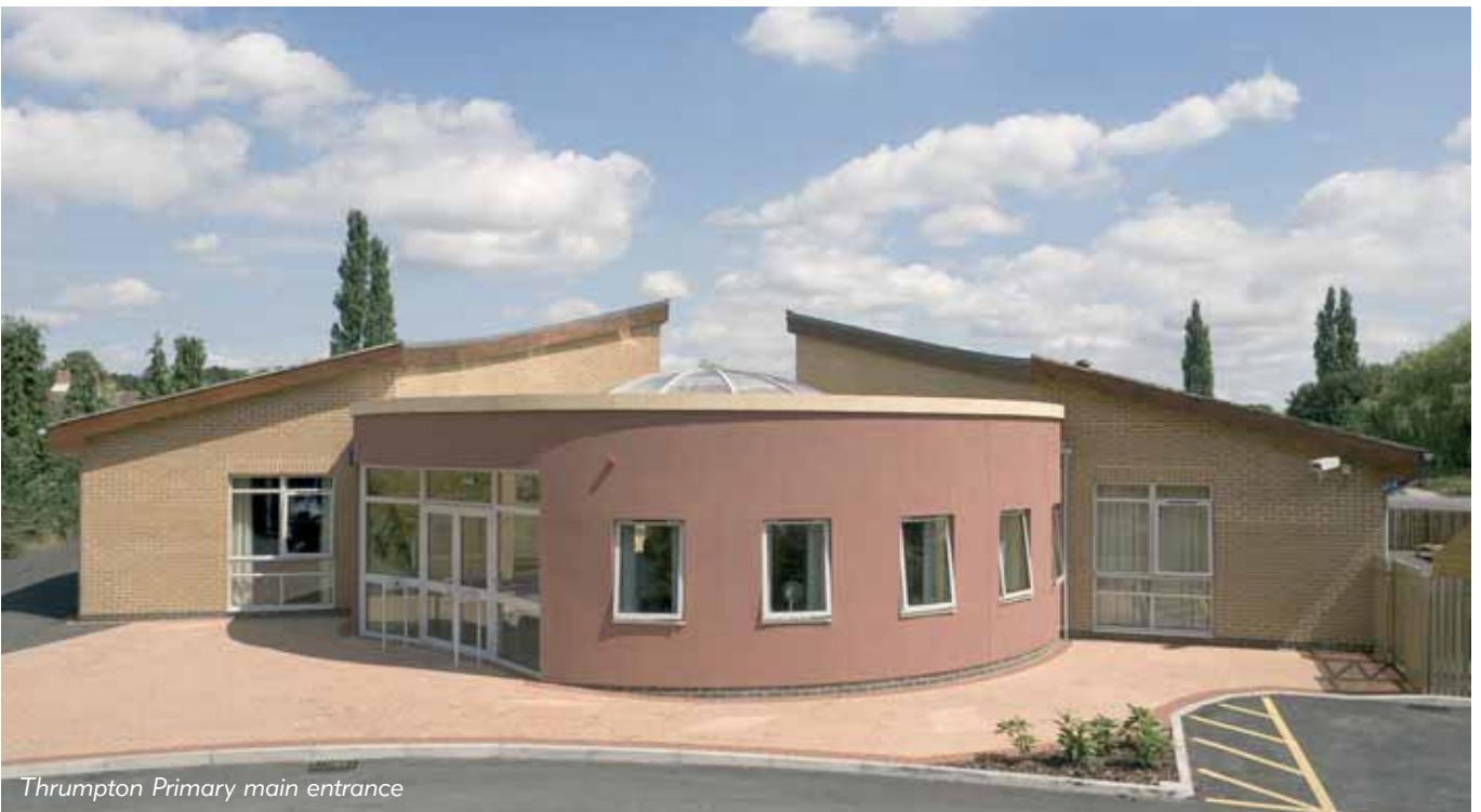
Thrumpton Primary Hall circular entrance
