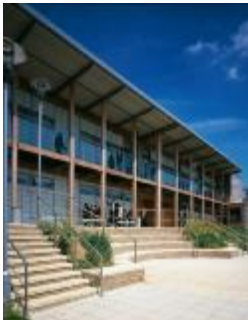
Highcrest Community School, High Wycombe
