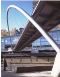
Churchill Way Bridge
