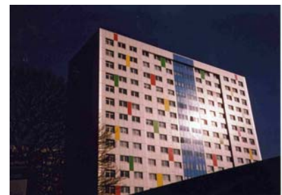
High Rise Flats, Anlaby Road, Kingston upon Hull.
