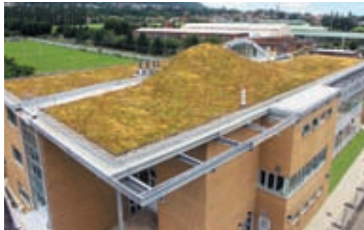
The sedum roof with 'eyelid' openings
