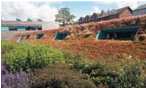
The Academy of St Francis of Assisi in Liverpool stimulated a new enthusiasm for education in its pupils, as well as achieving new standards of sustainable building design (Architects - Percy Thomas Partnership, now part of Capita).
