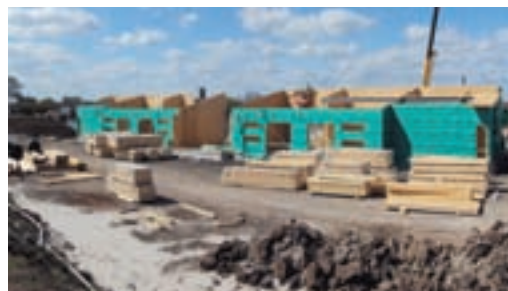
Installing the SIPS system on the ground beams
