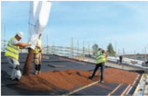
Laying the sedum roof
