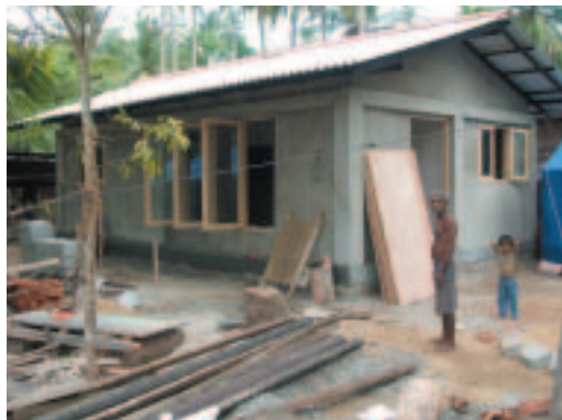
First house nearing completion
