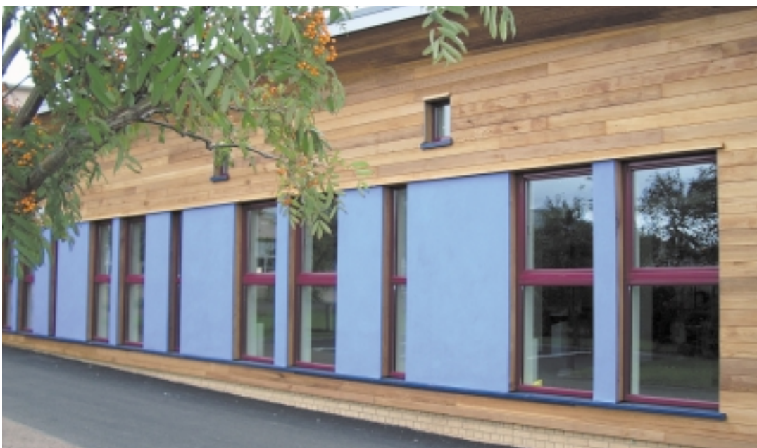
Extension to Dunbar Primary school dining area, using pre-fabricated Warmcell insulated Masonite panels
