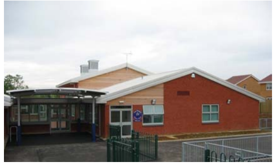
Photograph of a newly completed CLASP project at Kettering Primary School Architects, Northamptonshire County Council with Corstorphine and Wright Constructed by Skanska Integrated Projects under
