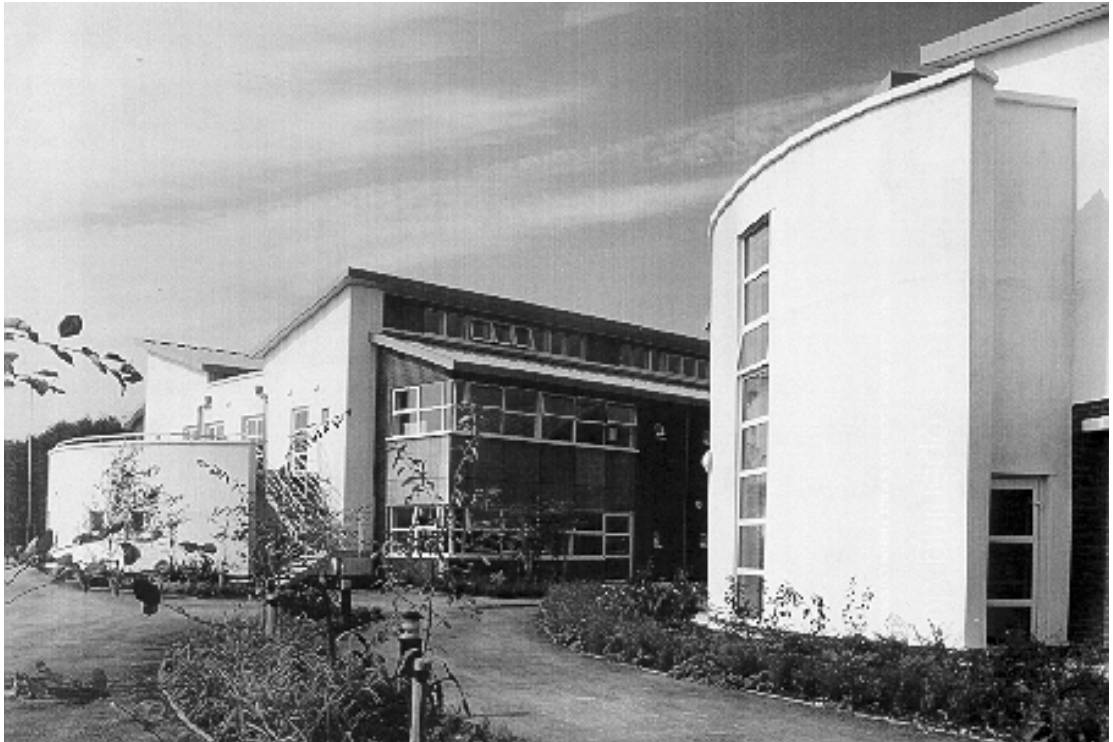
Colfox School at Bridport in Dorset cost £11.0m and was the first PFI funded school. Designed by Terence O'Rourke, Architects, and built by Jarvis Construction this successfully completed project was based on an output specification. The latest procurement methods seek to ensure even higher quality of design and construction through 'partnering' and other Egan style initiatives.
