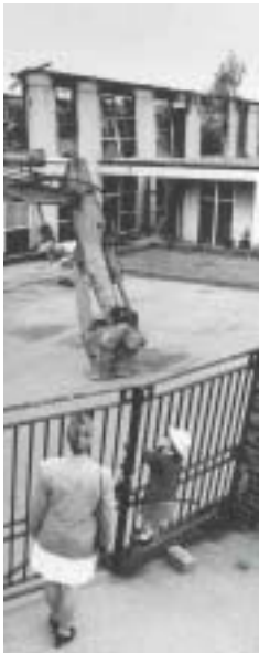
The result of a school arson attack
