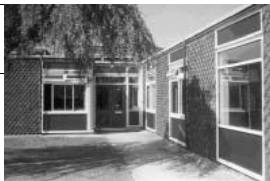
REPLACEMENT WINDOWS AT A NOTTS SCHOOL
