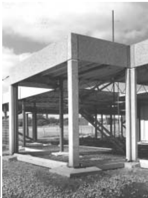
1960's PRE-CAST CONCRETE FOUNDATION
